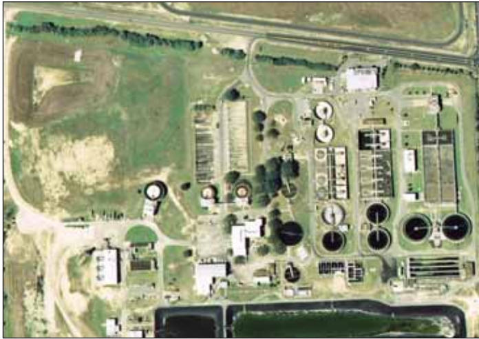
Aerial view of the 26.5-mgd Thomas P. Smith Water Reclamation Facility in Tallahassee, Florida.
