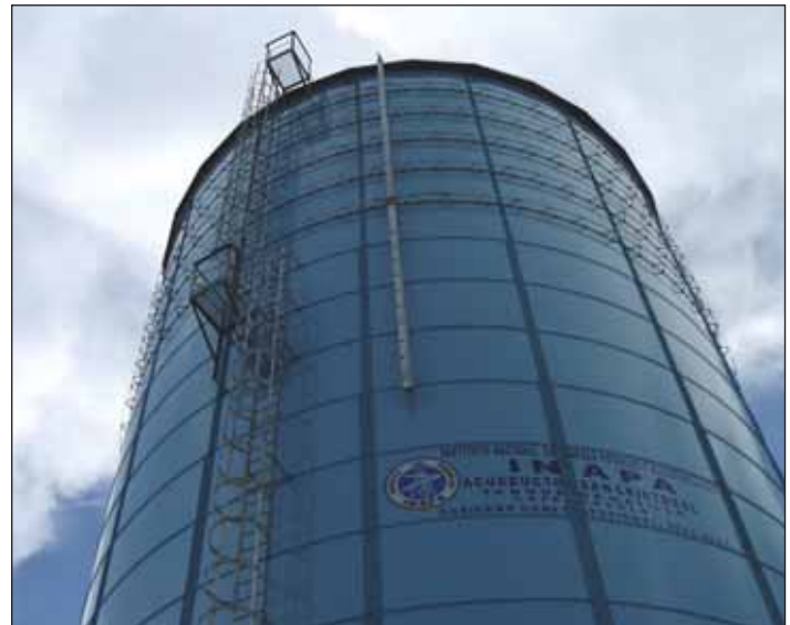
Hatillo water storage tank.
