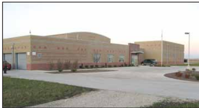
The porous pavement used in construction allows for gradual infiltration of stormwater through the soil, providing some natural water quality treatment and groundwater recharge.
