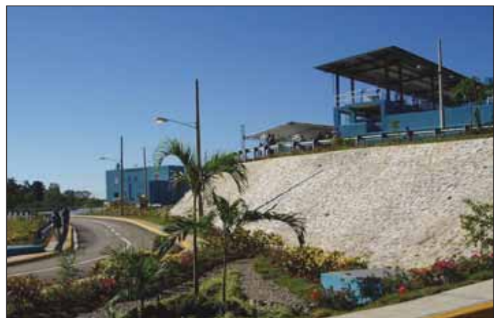
San Cristobal Water Treatment Plant.
