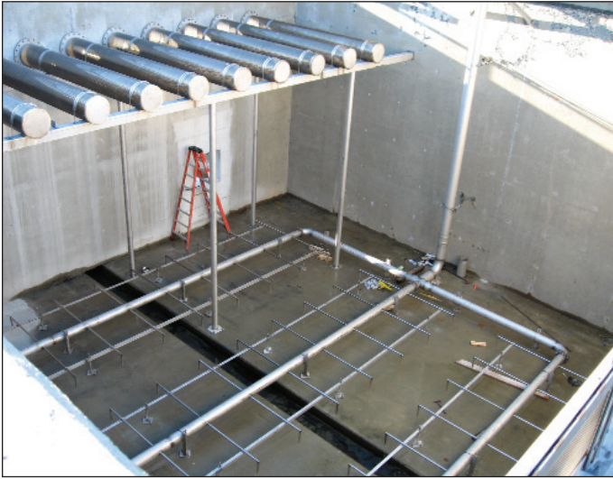
Free floating media for IFAS systems are retained by submerged wedgewire screens, increasing the capacity of the activated sludge system in the same tank volume.
