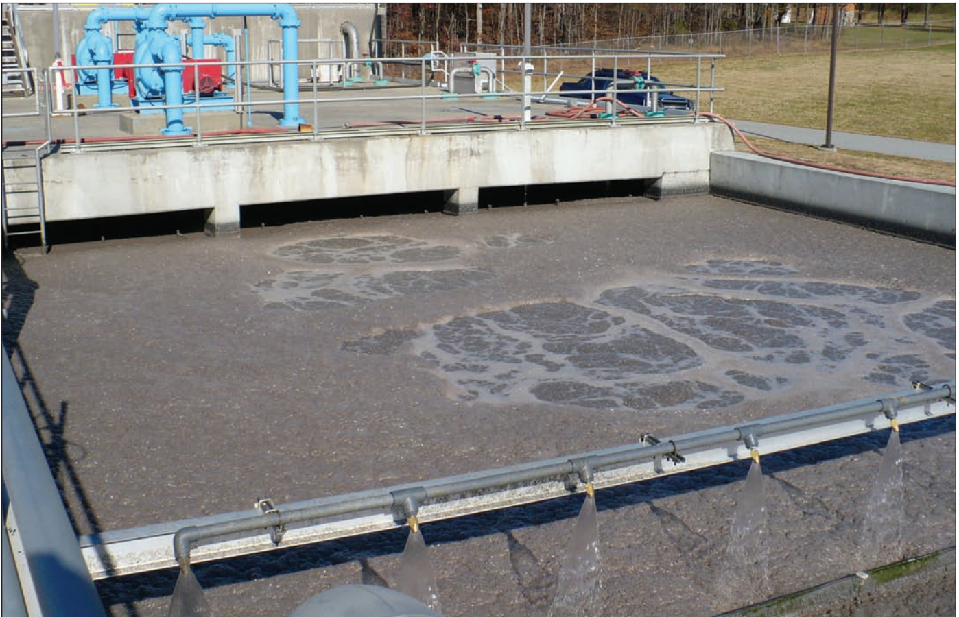
Free floating media for IFAS systems are retained by submerged wedgewire screens, increasing the capacity of the activated sludge system in the same tank volume.
