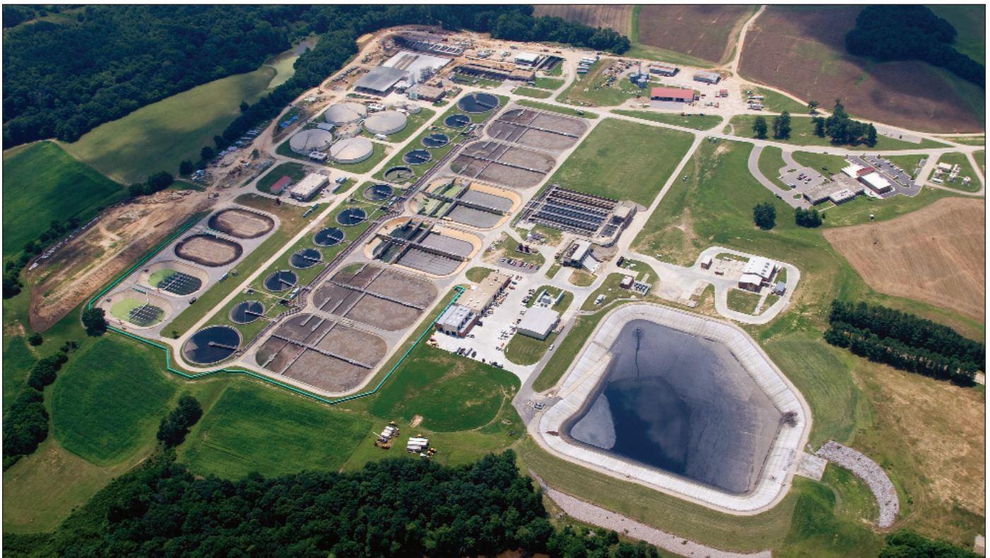
The Neuse River Wastewater Treatment Plant is currently the largest wastewater treatment facility meeting “Limits of Technology” TN limits on the East Coast.
