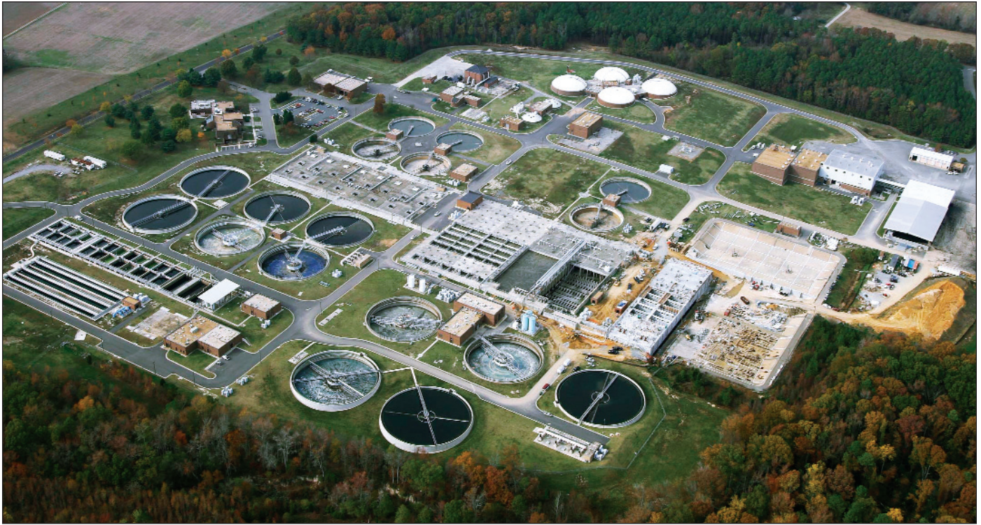
Optimization and a change in carbon source at the Henrico County Water Reclamation Facility has resulted in a chemical savings of $400,000 per year.
